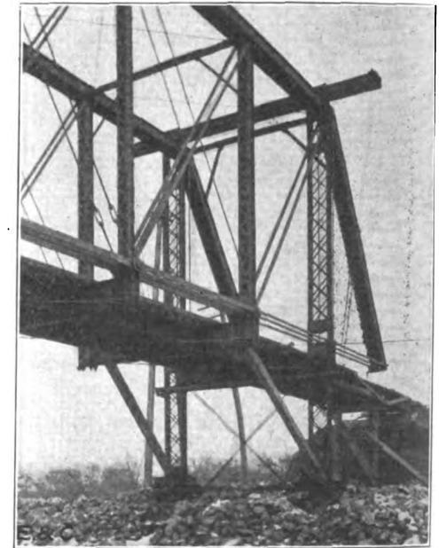
Fig. 2. View of End of Span, Showing Details of Construction Used to Support Span During Reconstruction of Abutments.
