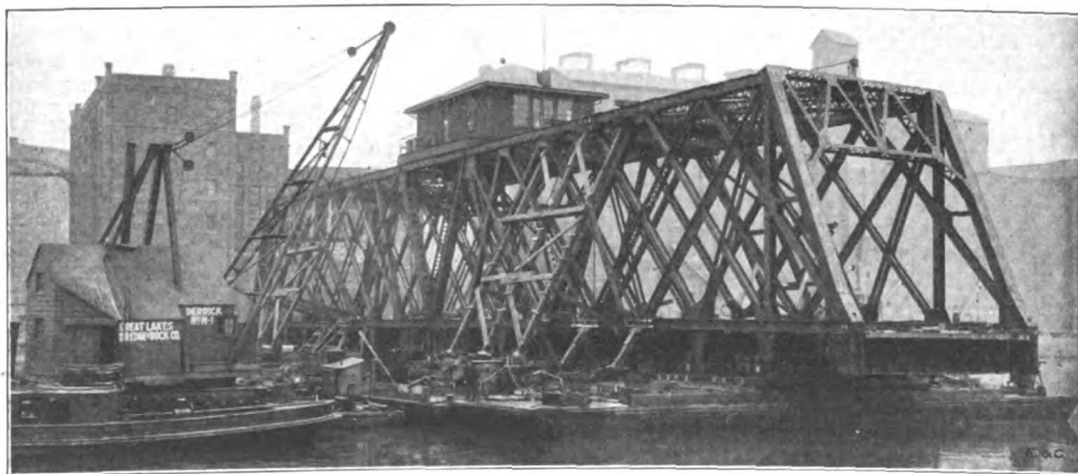
Fig. 1. View Showing New Double-Track Swing Span on Scows—Note Struts Used to Distribute Loading—C. & N. W. Ry. Bridge, Milwaukee, Wis.
